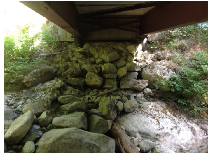
Left Bank Abutment when facing downstream
