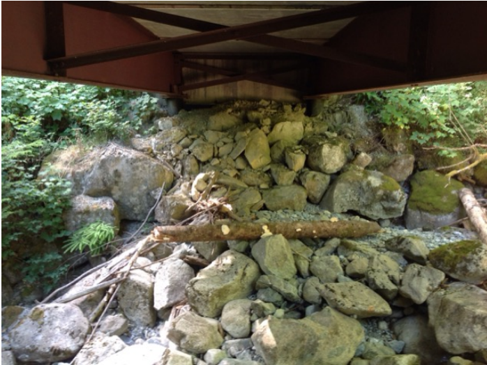
Right Bank Abutment when facing downstream
